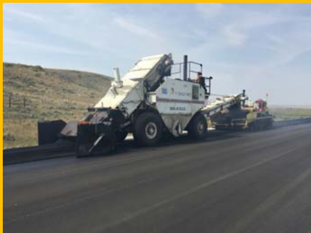
2. APPLIED A 4" LIFT OF HOT PLANT MIX
