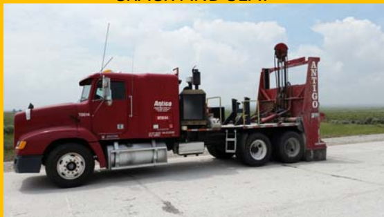
•CRACK AND SEAT THE MILLED SURFACE OF THE CONCRETE TO LIMIT REFLECTIVE CRACKING
