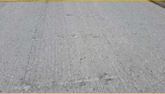
3" MILLING CONCRETE PAVEMENT
