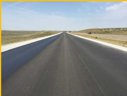
1. APPLIED AN INITIAL LIFT OF 1" OF LEVELING HPM
