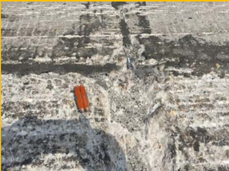
3" MILLING CONCRETE PAVEMENT
